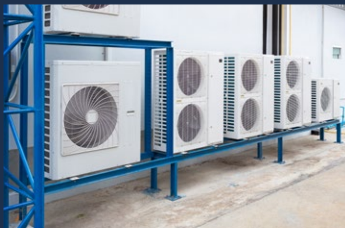
REFRIGERATED AIR HANDLER / CONDENSING UNITS
